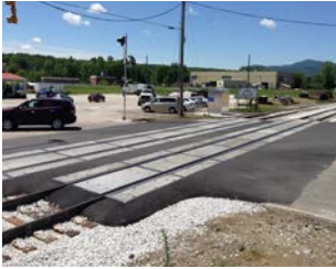
Rutland West Street grade crossing (before and after)
